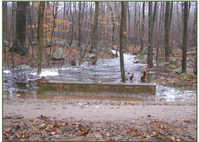
Right. Photo looking upstream from the culvert crossing flooding and road overtopping causing erosion and sedimentation impacts to Mott Hill Brook.
